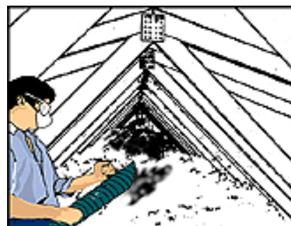
Blown-in attic insulation
